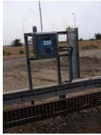
4 x TTC-1 controller with 7767 Zener barriers, wired to junction boxes with branch connectors local to the tanks.
