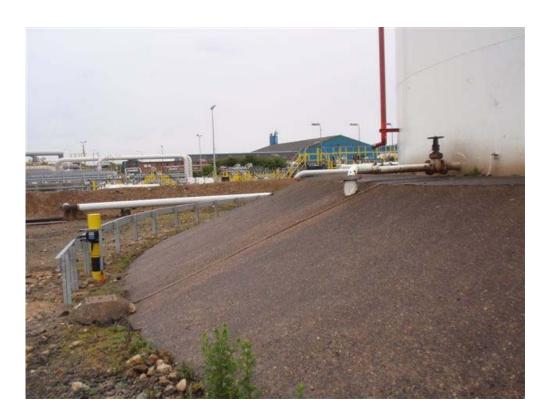
TT-FFS-100-3-L attached to the base of a post within the bunded area around the base of the tanks. Exe junction box housing terminals for the connection of the FFS.
